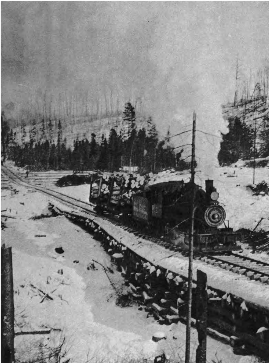
Blasting up a steep grade, a Duluth and Northeastern engine moves one flat of logs at a time, as steam jammer at the end of the spur loads another car. Unballasted track and fill work in the deep cut were typical on these temporary spurs.
