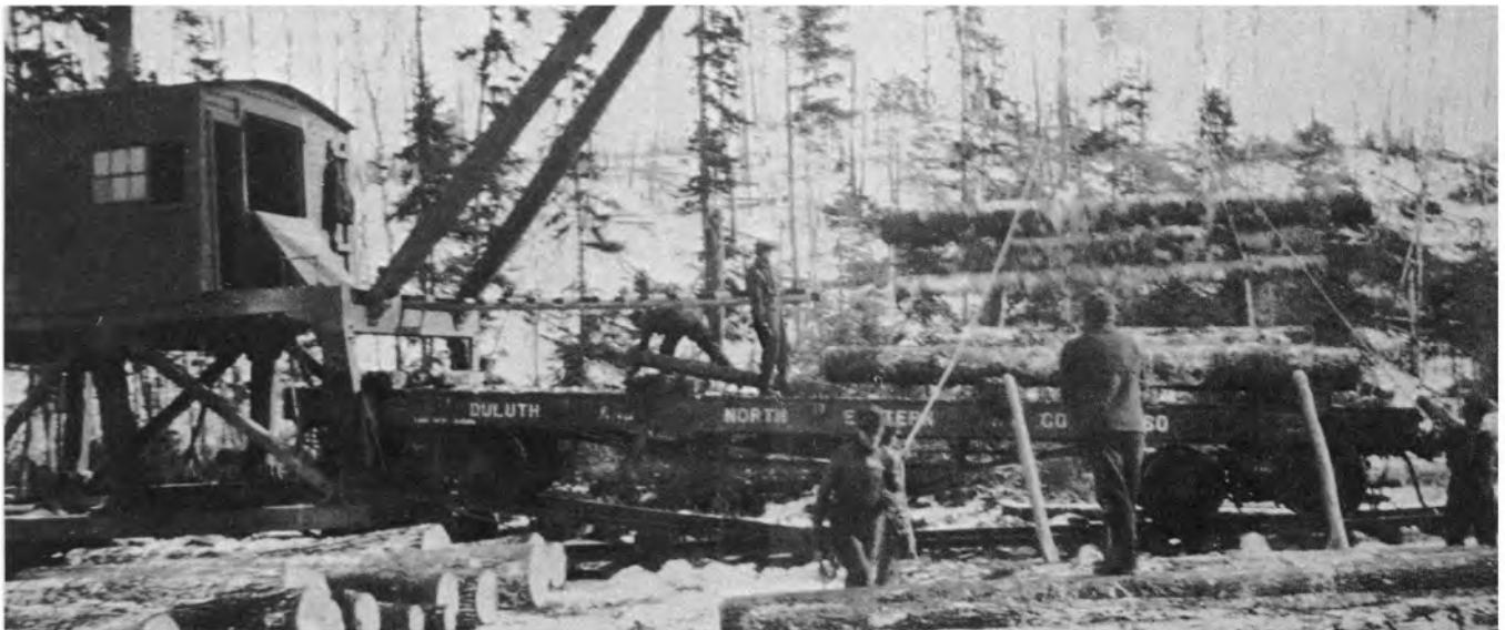
Steam jammer pulled flatcars through as it loaded them. A good crew loaded 16 cars a day.
