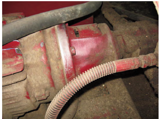
This photo shows the near miss at a sawmill involving a hydraulic unit where the coupler housing was the area of concern between the electric motor and the hydraulic pump. The fire was contained inside the coupler housing.
