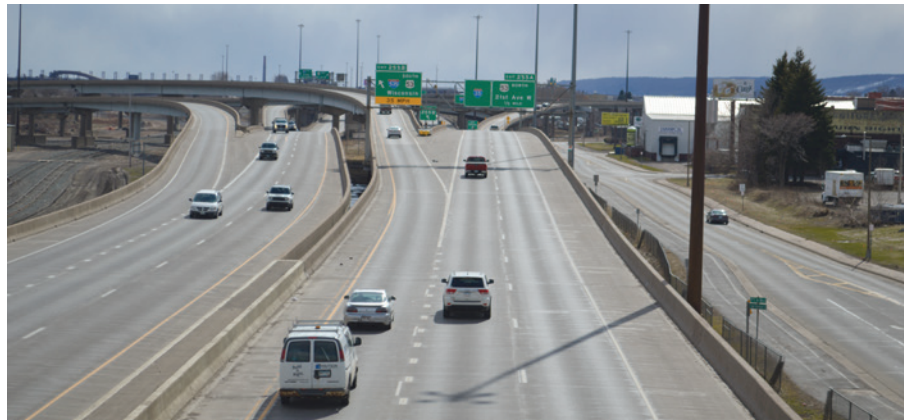
Site of MnDOT’s Twin Ports Interchange project in Duluth, now scheduled to begin in 2021.
