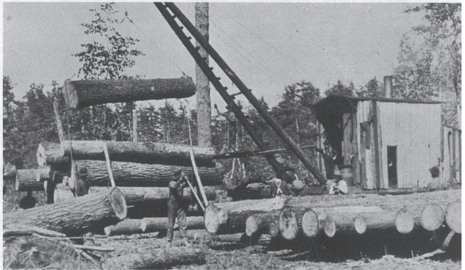
Operating from a flat car, the steam jammer above loads small Russell cars. The slide ass jammer below was moved along the tops of the cars; this type was much used along the M. & I. Railroad by Crookston and International Lumber Co.
