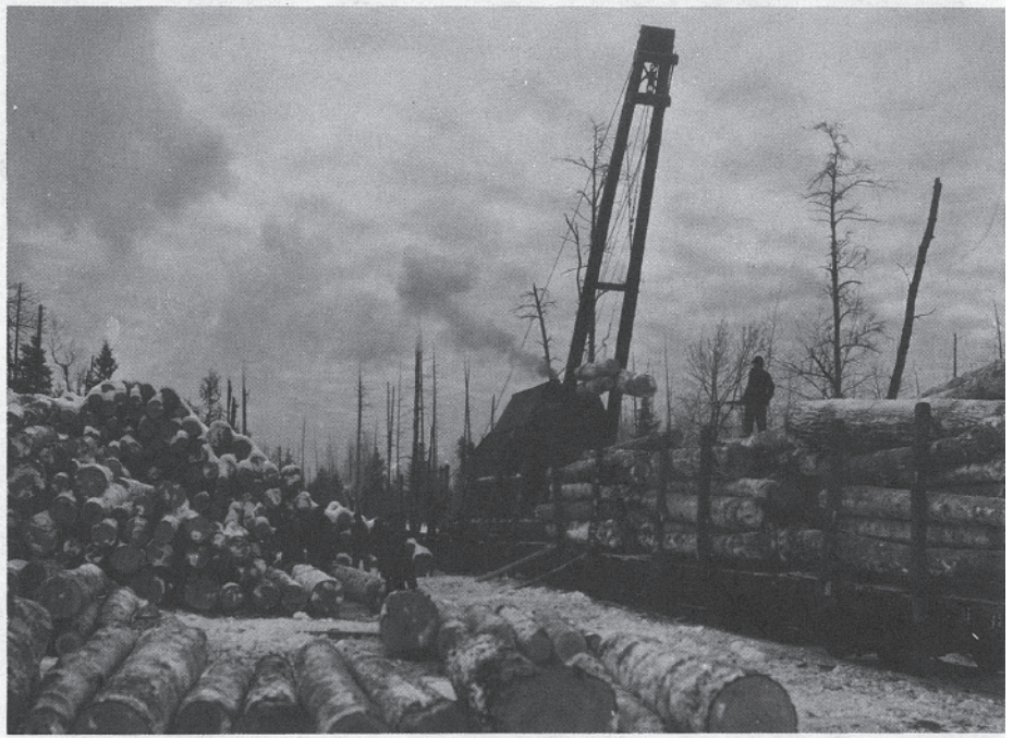
Operating from a flat car, the steam jammer above loads small Russell cars. The slide ass jammer below was moved along the tops of the cars; this type was much used along the M. & I. Railroad by Crookston and International Lumber Co.
