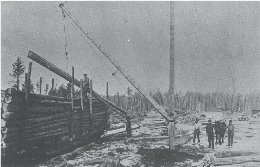
The swinging boom "jin pole" above was the type used in cedar yards. Below is a good view of woods jammer showing cross chains and the three blocks—one on top, one at bottom, and traveling block. Jammer could tilt over center of sleigh.
