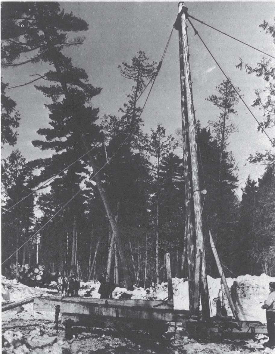
The swinging boom "jin pole" above was the type used in cedar yards. Below is a good view of woods jammer showing cross chains and the three blocks—one on top, one at bottom, and traveling block. Jammer could tilt over center of sleigh.
