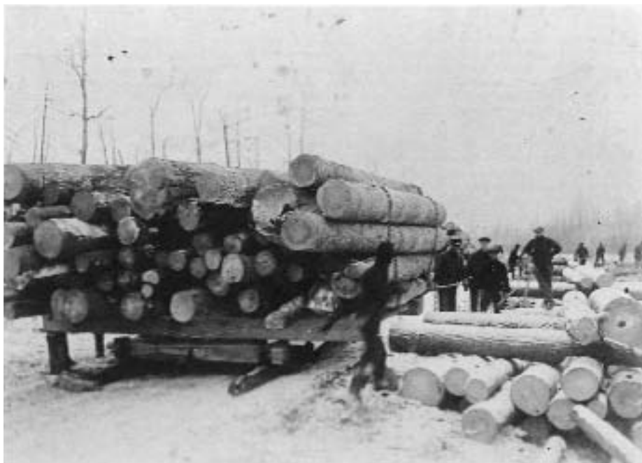
Load of logs about were photographed on Oliver Mining Co. operations at In-on Lake near Bemson. The 14-inch trucks on the right were hewn with a broad axe by a wood butcher. The jaw saw below was constructed entirely by a wood butcher— even to going into the woods to select the logs. Sledges in the foreground also were built by wood butchers in camp. Note the "rustent stakes" with built-up holes. Brier Ryan photos.
