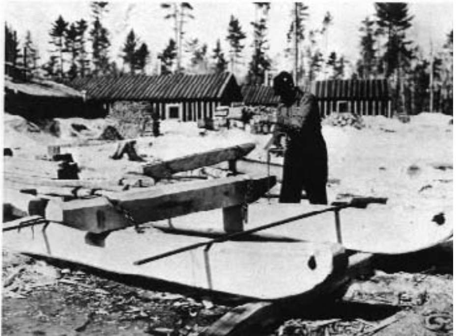
In a logging camp south of International Falls about 1910, a wood butcher builds a two-hank dry, mostly of birch. The go-devil used for skidding a pine log below was made in camp by a wood butcher. Minnesota Historical Society photo.
