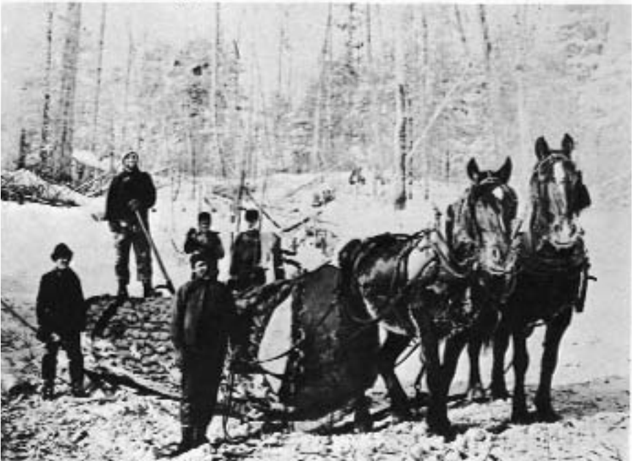
In a logging camp south of International Falls about 1910, a wood butcher builds a two-hank dry, mostly of birch. The go-devil used for skidding a pine log below was made in camp by a wood butcher. Minnesota Historical Society photo.
