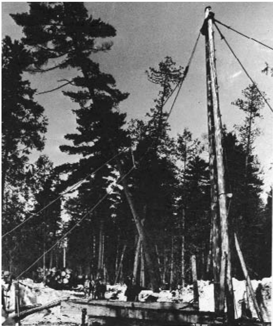
Load of logs about were photographed on Oliver Mining Co. operations at In-on Lake near Bemson. The 14-inch trucks on the right were hewn with a broad axe by a wood butcher. The jaw saw below was constructed entirely by a wood butcher— even to going into the woods to select the logs. Sledges in the foreground also were built by wood butchers in camp. Note the "rustent stakes" with built-up holes. Brier Ryan photos.
