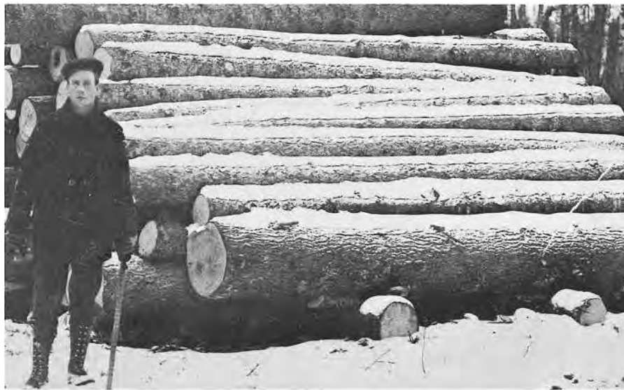
Above: Clyde Johnson, a state scaler in the Big Fork area, 1917. Below: Dan O'Connor looks over a defective log; logs like this called for experienced scalers.
