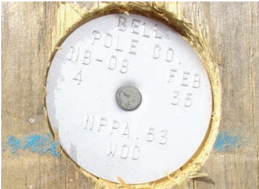
An aluminum tag is placed on each finished pole for identification purposes.
