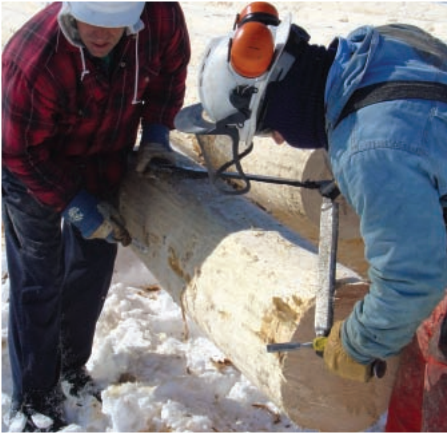
Workers at the Barron facility remove bark by hand that wasn't removed by the peeler.
