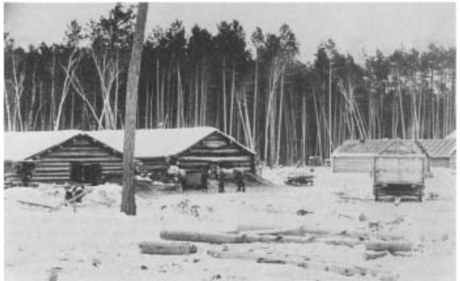
Early camp scene (top) shows barns and water tank. The camp foreman checked his roads and work crews daily. Note the oxen used in cross haul loading (bottom).
