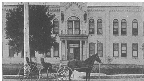
St. Vincent’s Hospital, Crookston
