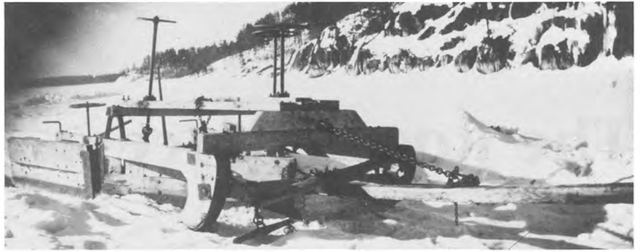
Right: rut cutter used in making ice roads, with top wheels to adjust cutting blades and bottom wheels to set V-plow and wings. Below: water tank with loading barrel on top. Bottom: a load of 56 picked logs—37,120 board feet.
