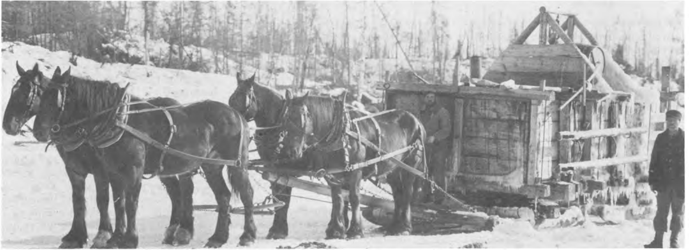
Right: rut cutter used in making ice roads, with top wheels to adjust cutting blades and bottom wheels to set V-plow and wings. Below: water tank with loading barrel on top. Bottom: a load of 56 picked logs—37,120 board feet.
