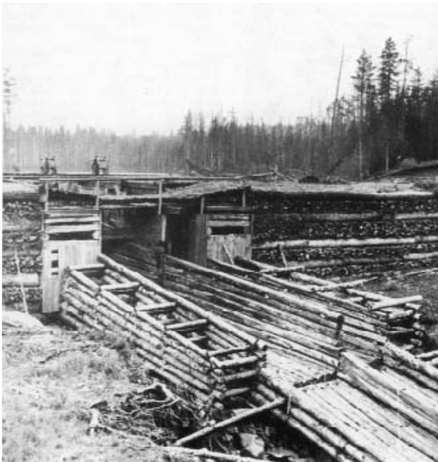
This large log driving dam is constructed of timber from the nearby woods. Its brush layered into the dam helps hold the fill from washing out. One man could open the gates with winches atop the dam.
