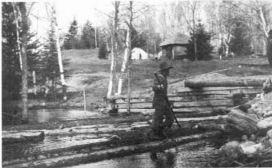
These river drivers poled logs toward dam gates and the "log shoots" leading downstream.
