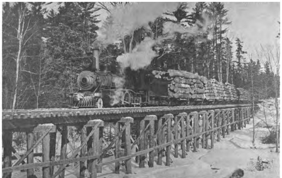
A trainload of logs on the Alger Line out of Knife River crosses the long trestle over McCarty Creek.
