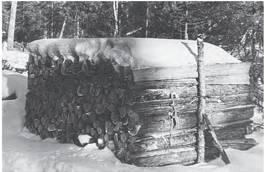
Lagging for mines (above) was cut in six-foot lengths and split in the woods.
