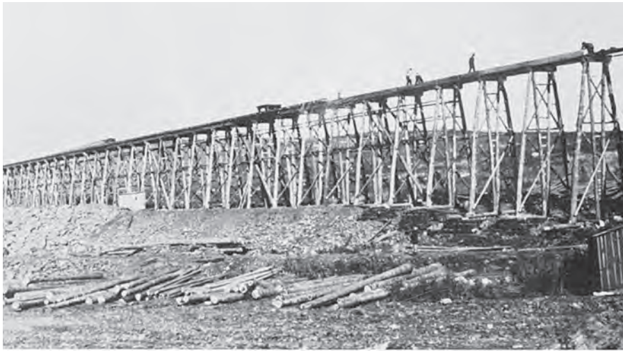
Trestles built of round timber were sometimes a half mile long. Tall Norway pine was used for trestle logs.
