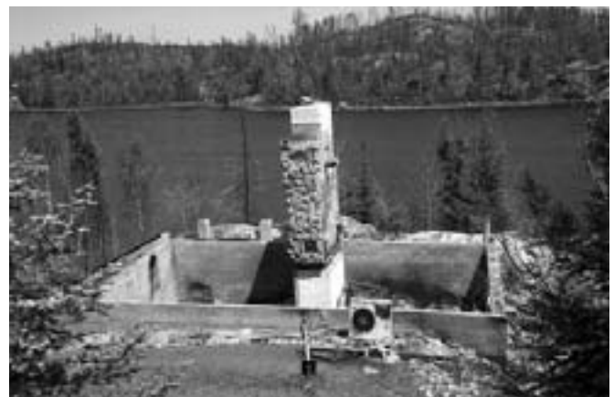
All that remains of this lakefront house are the foundation, fireplace, and air conditioning unit.
