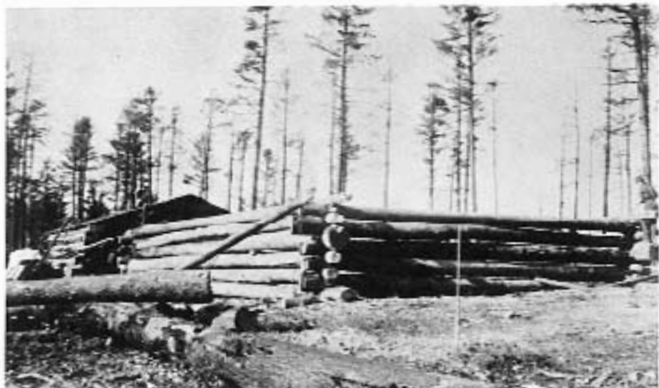
Most early camps were made of logs, as this one under construction.
