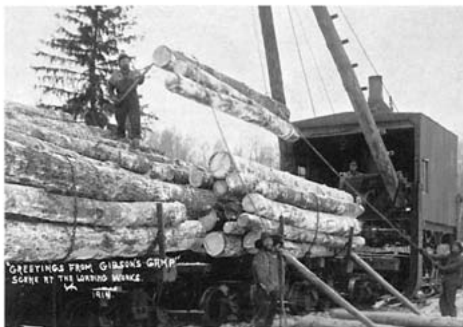
Loading logs onto Russell cars using a steam jammer.
