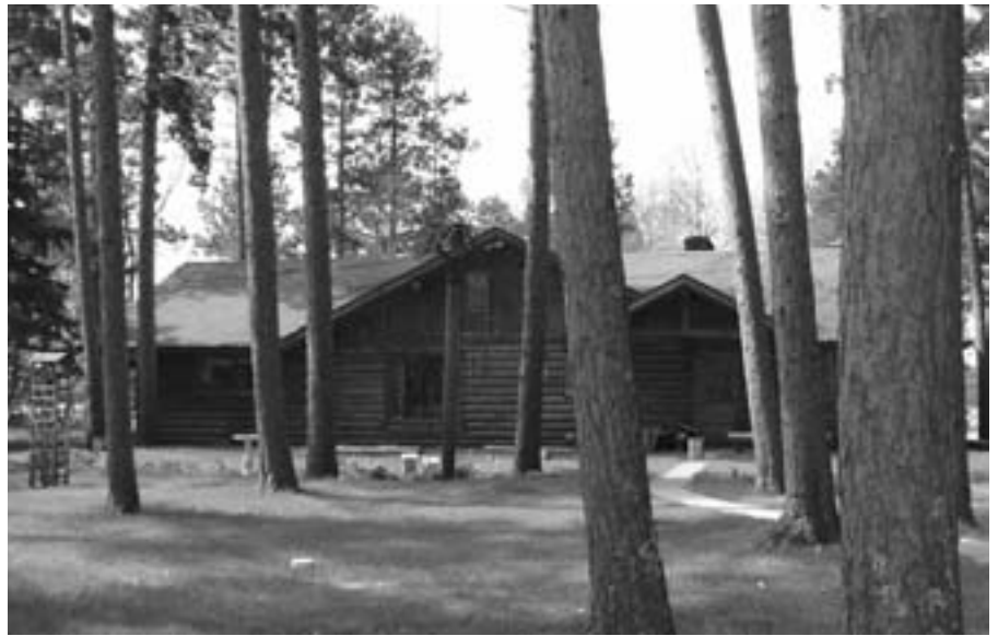
The original home Burgess Bach built on Lake Kabekona.
