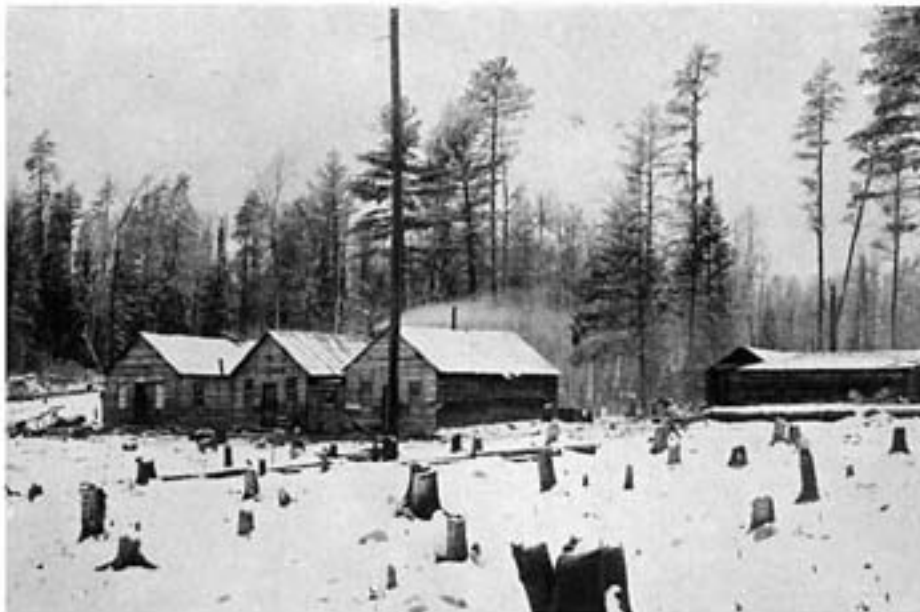
Logging camp about 1892. Most camps of this era were made of logs
