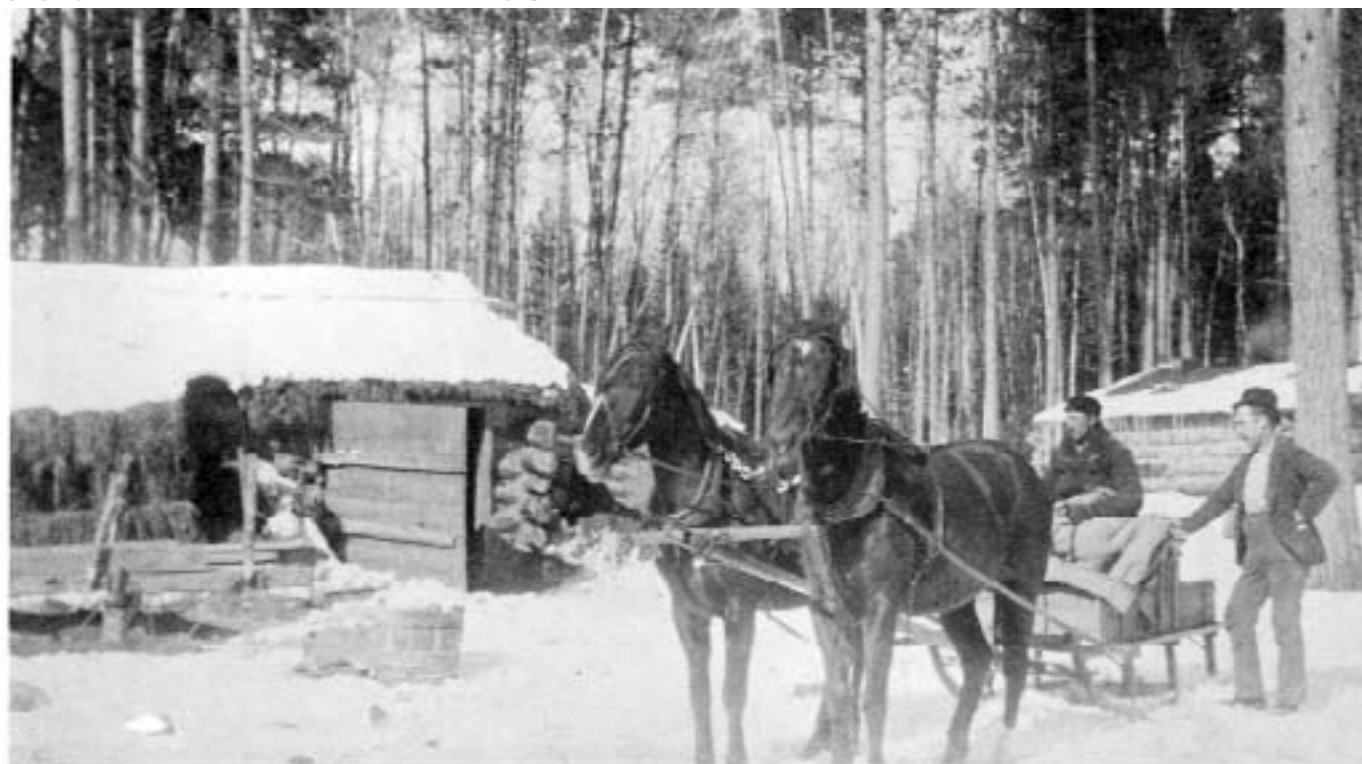
A tie team moved this "walker" between Duluth & Winnipeg Railroad camps.
