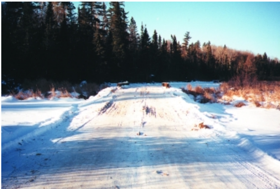
Temporary bridge installed over Little East Creek.
