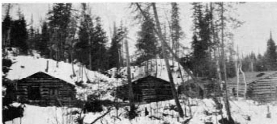
Top photo: A small pioneer camp, all buildings of logs. Center: Camp cook, his helpers, clerk, camp foreman, bull cook and "washing boys" were six of this group. These the light sleds used by the walking boys to travel from camp to camp. Bottom: Splitting wood for the bunkhouse, the bull cook always found a good supply at hand.
