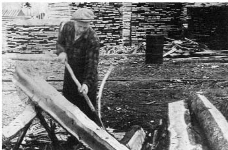
Peeling ties with a spud (above). All ties were peeled with a spud rather than peeling knives. Below: one of the smaller skiffs that moved ties on "rough" roads.
