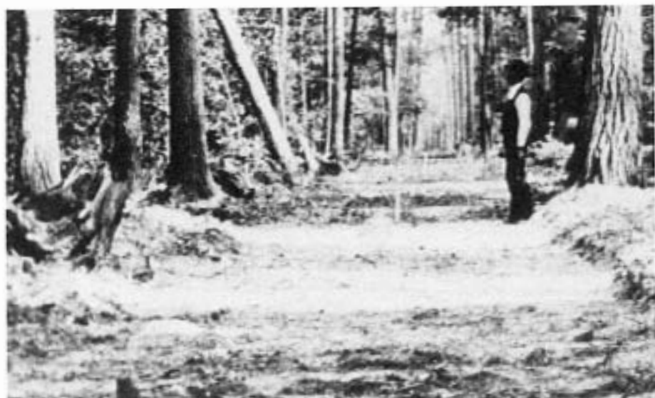
Ties and rails are ready to be laid on this railroad spur through the timber. Below. Temporary or "skidder" tracks are laid on the surface, with no ballast.
