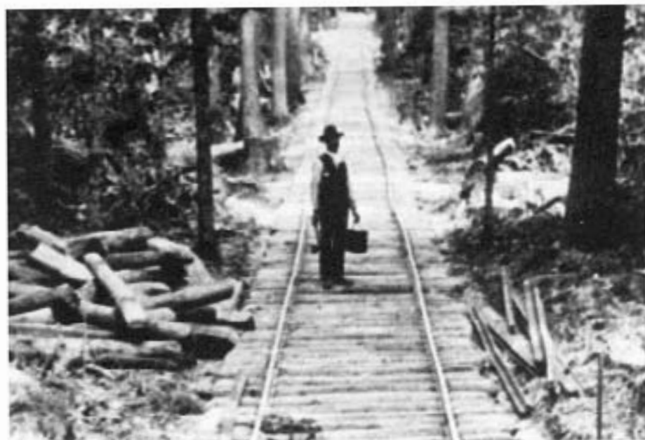
Ties and rails are ready to be laid on this railroad spur through the timber. Below. Temporary or "skidder" tracks are laid on the surface, with no ballast.
